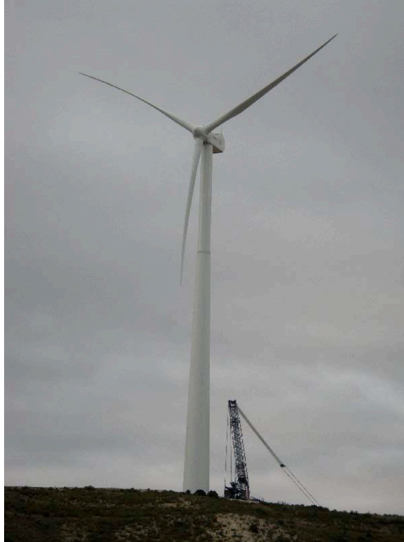
Figure 1. Mixed 80 m concrete and 40 m steel tower
