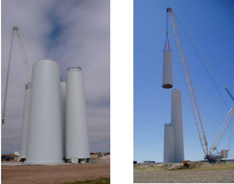
Figure 2. Assembling of tower segments obtained from precast elements
